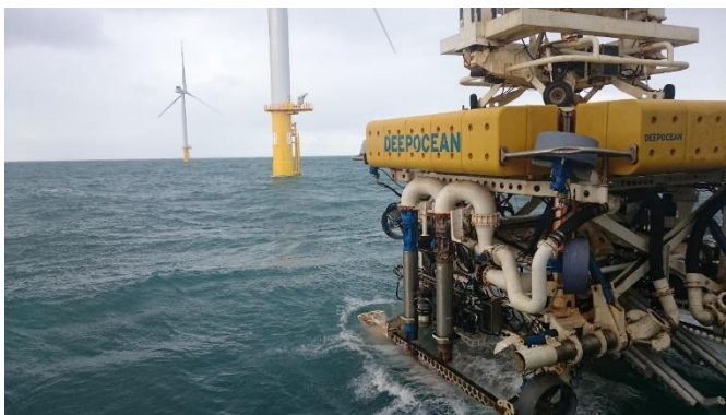
Plate 2 - Jet trencher (image courtesy of DeepOcean)
